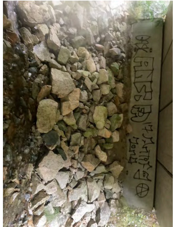
Right Bank Abutment when facing downstream
